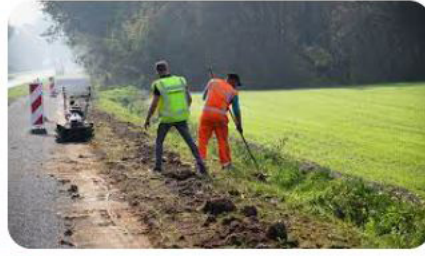
Hogenhout Infratechniek Over Ons | Hogenhout Infrate...
